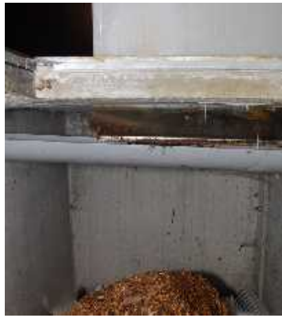
Checking urine gutter
